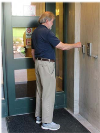
Card Access Reader on Exterior of Building
