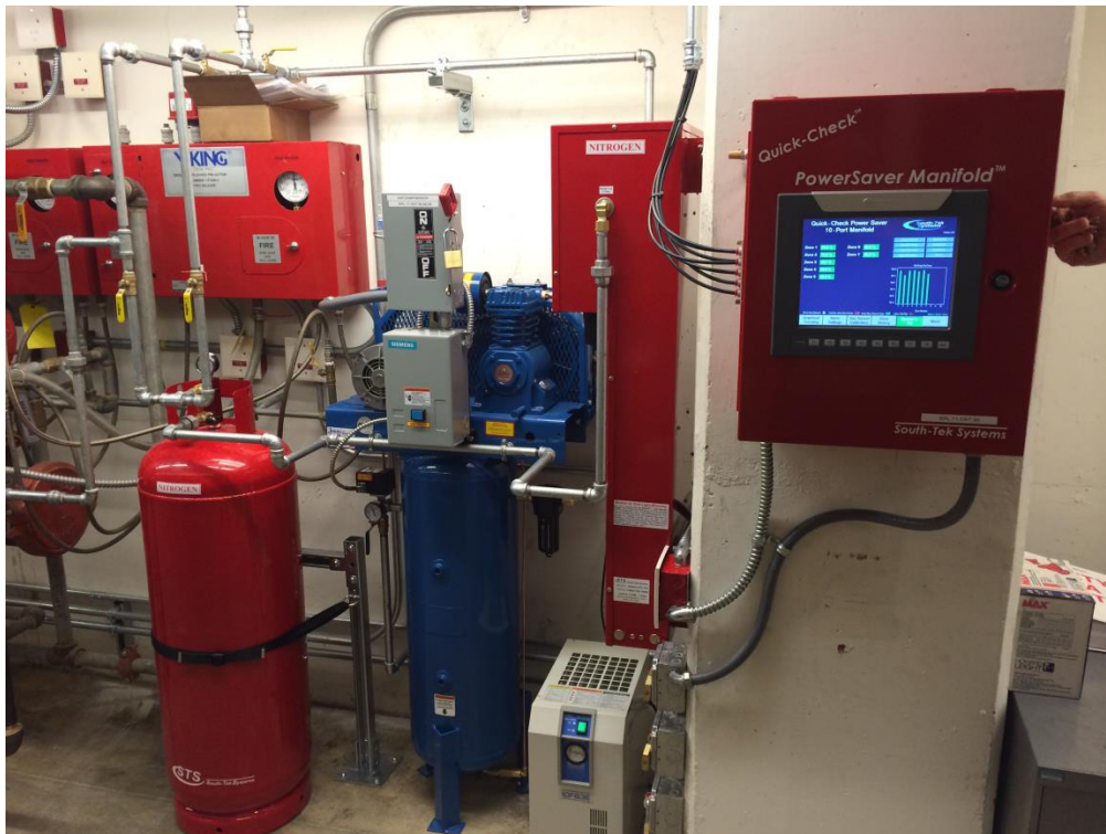
Photograph of a nitrogen generator system currently in service at the Virginia Museum of Fine Arts.
