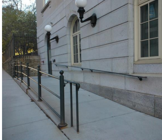
Figure 2 – Dimension ramp with slope less than 1:12
